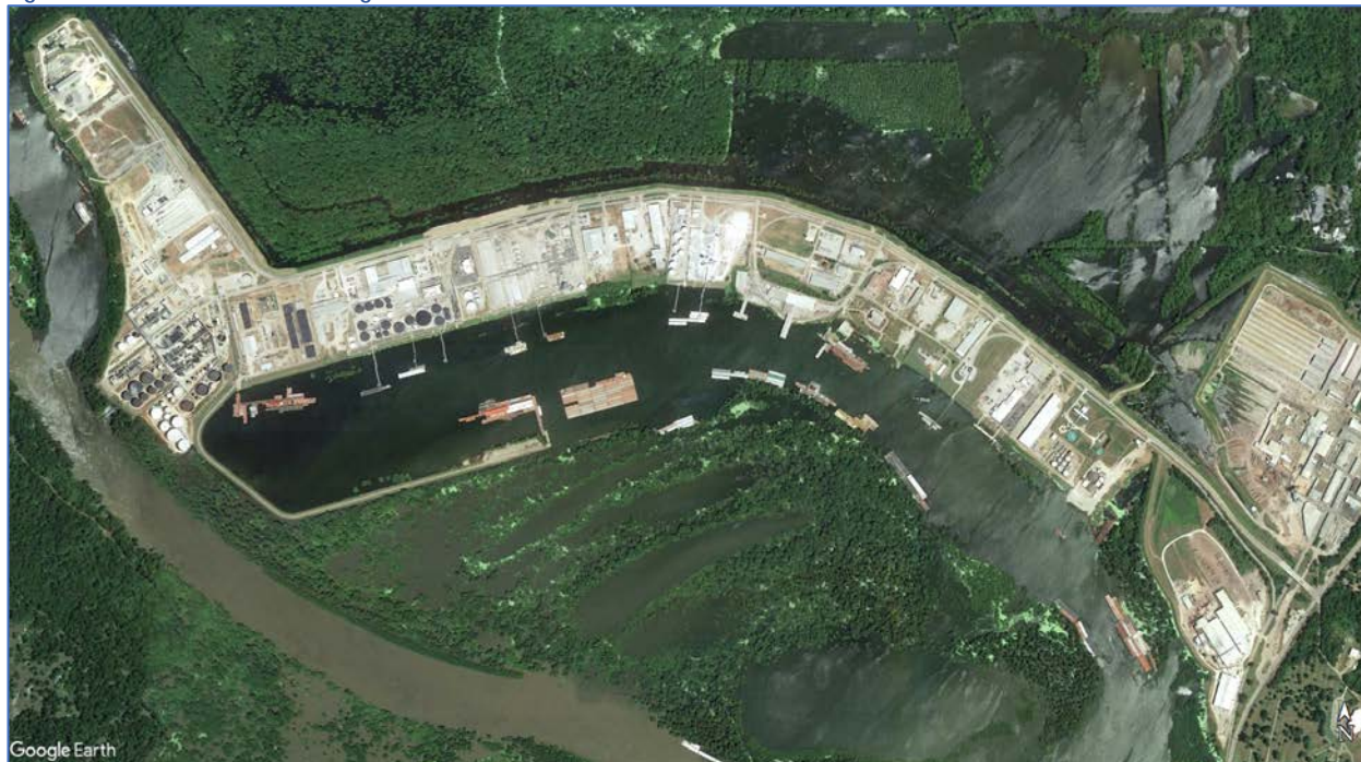
Figure 14 View of Port of Vicksburg Public and Private Terminals
